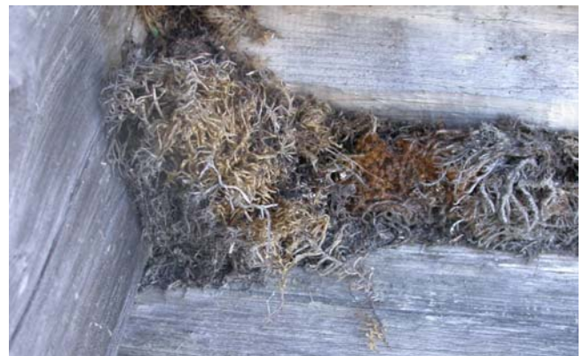
Figure 2. Moss chinking in a fishery hut on the dock near the Rock Harbor Light House, Isle Royale National Park, Michigan, USA. Photo by Diane Lucas.
