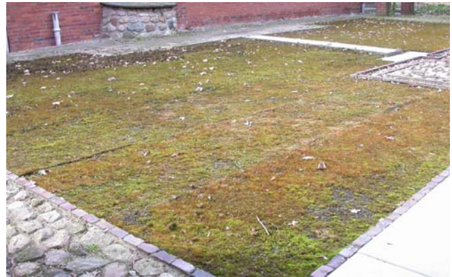
Figure 12. This completed green roof has a formal design, but many are more casual. Photo by Jan-Peter Frahm.
